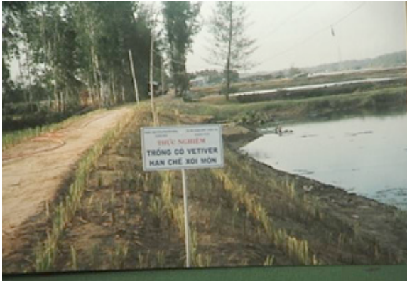
Rural road batter stabilisation (brackish water)
