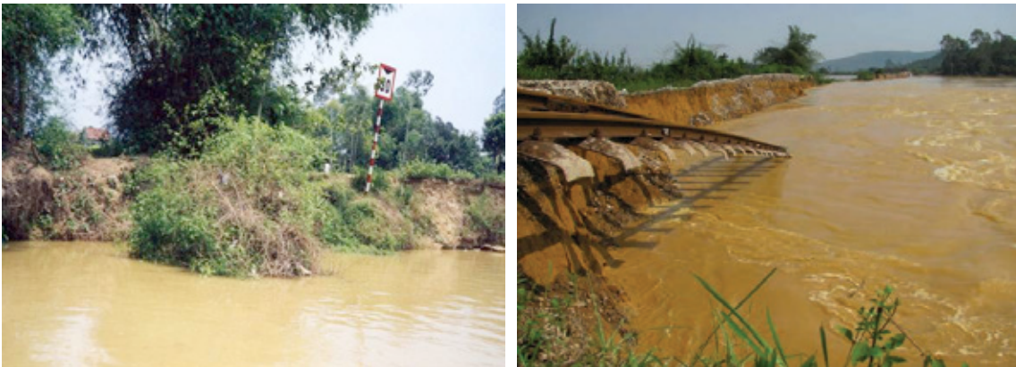
Annual flash floods cause several damages to dikes and rural roads
