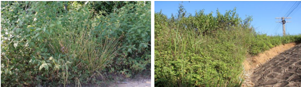
Invasion of weeds due to lack of maintenance causing over shading
