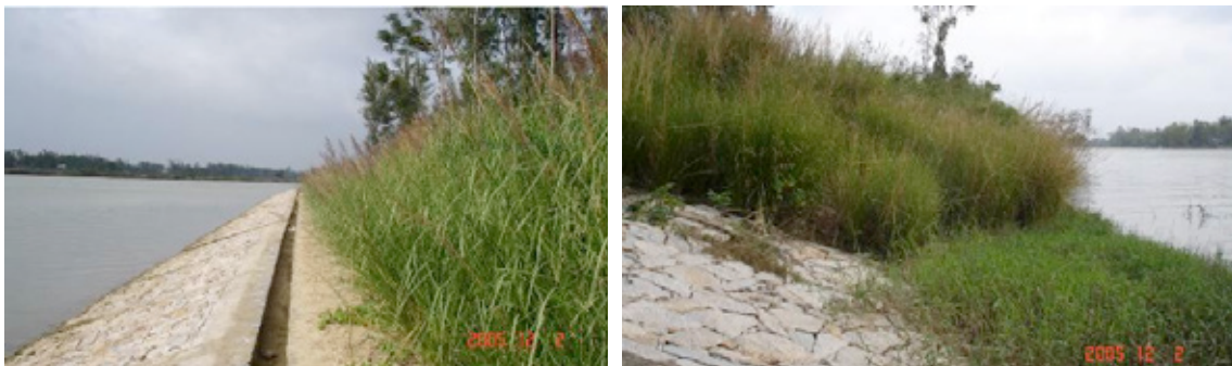
Vetiver protects An Luu Embankment
