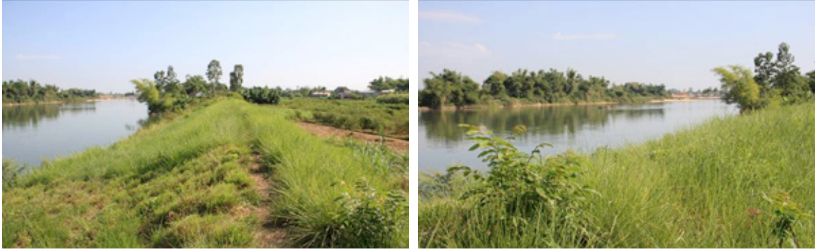
A highly effective & successful section of a freshwater river where is was properly maintained
