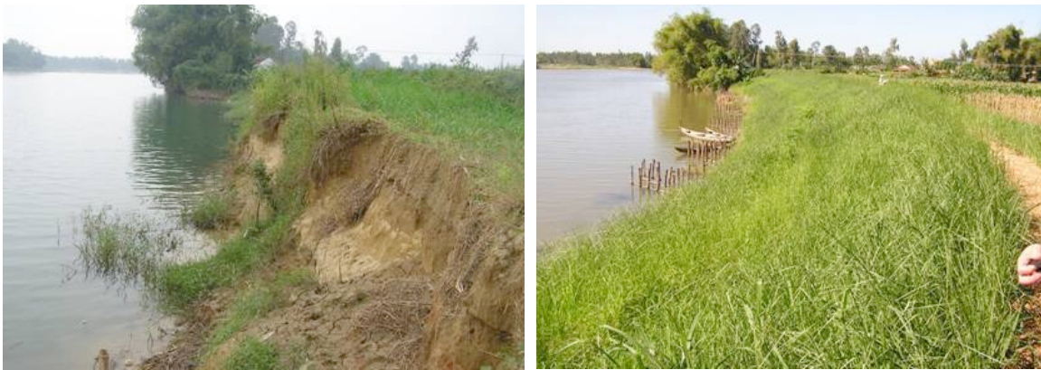
Small river bank stabilisation (brackish water)
