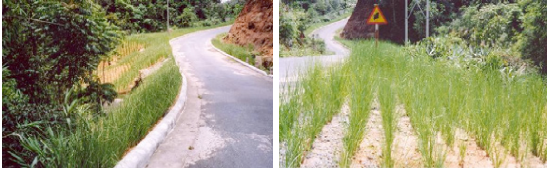
Slope stabilization at Ba Na road
