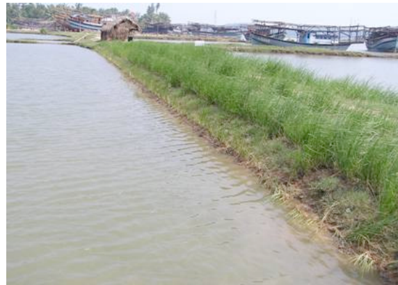
Prawn farm dike batter stabilisation (brackish water)
