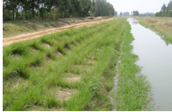
Canal bank stabilisation (fresh water)
