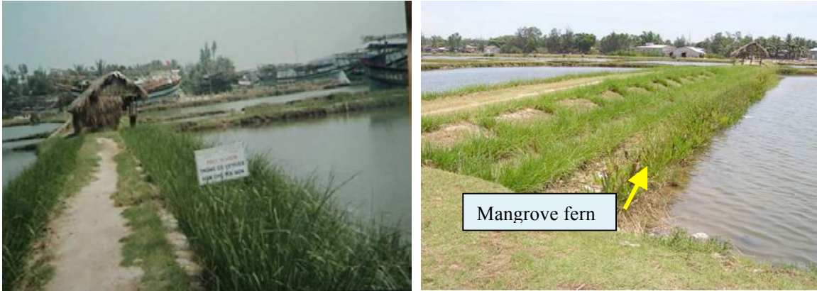
To protect the toe of the batter from brackish water inundation, planting of mangrove fern or local salt tolerant plants is recommended
